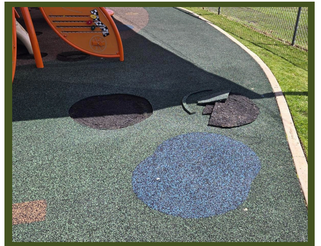
YELLOWJACKET POURED IN PLACE REPAIRS
